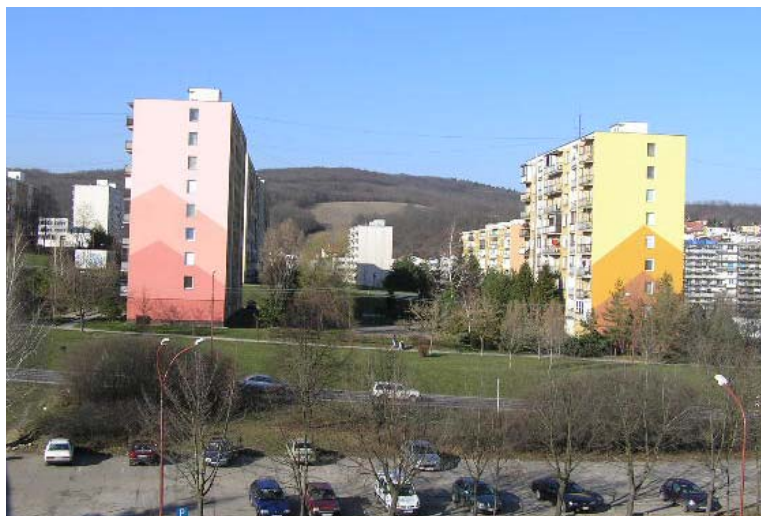
Figure: Example of block of flats type “T 06 B” after heat insulation of gable walls.
