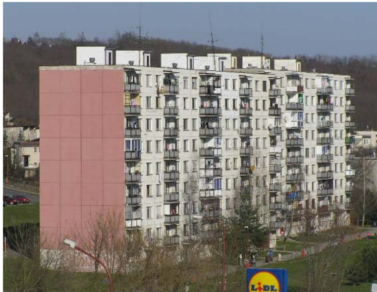
Figure: Example of block of flats type “T 06 B” – previous state.
